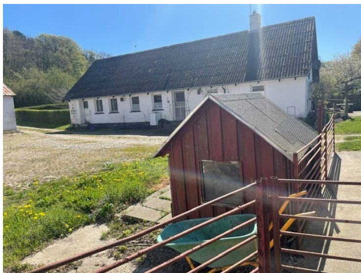
Beboelse under renovering - front
