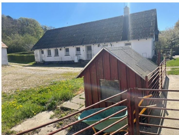
Beboelse under renovering - front
