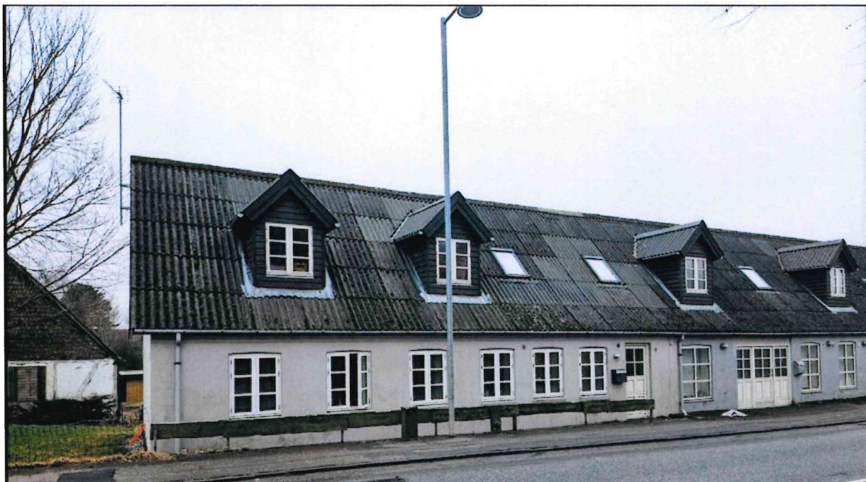
Facade mod nord (mod Rudsgade)
