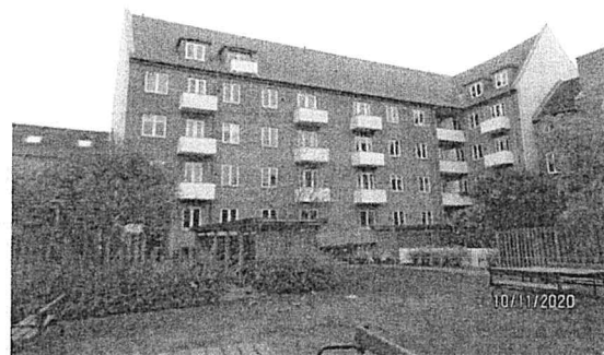
Altaner, facade mod baggård
